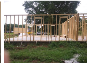
HOUSE #4: Framing has gone up! on HOUSE #4
