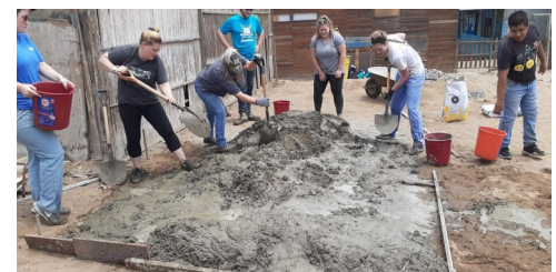
Building a classroom!
